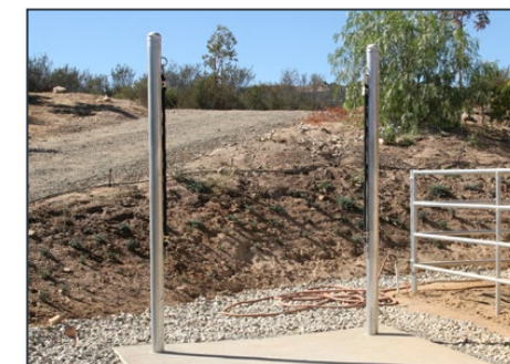
Cross Tie Posts
