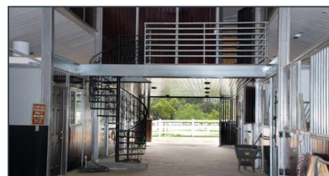
FCP Steel Mezzanine
