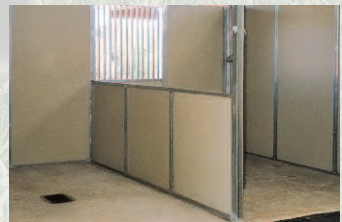
Wash Divider Wall
