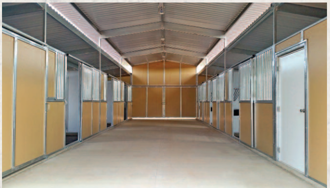
Interior View – 16' Breezeway Raised Center Aisle Barn
