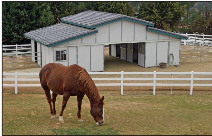
RCA barns provide increased ventilation and natural light.
